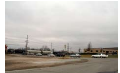
The at-grade train crossings cause backups and deter business
