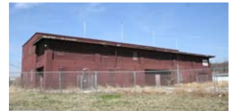
This old concrete structure still flies the flagpoles from the original Riverside Park Jockey Club.
